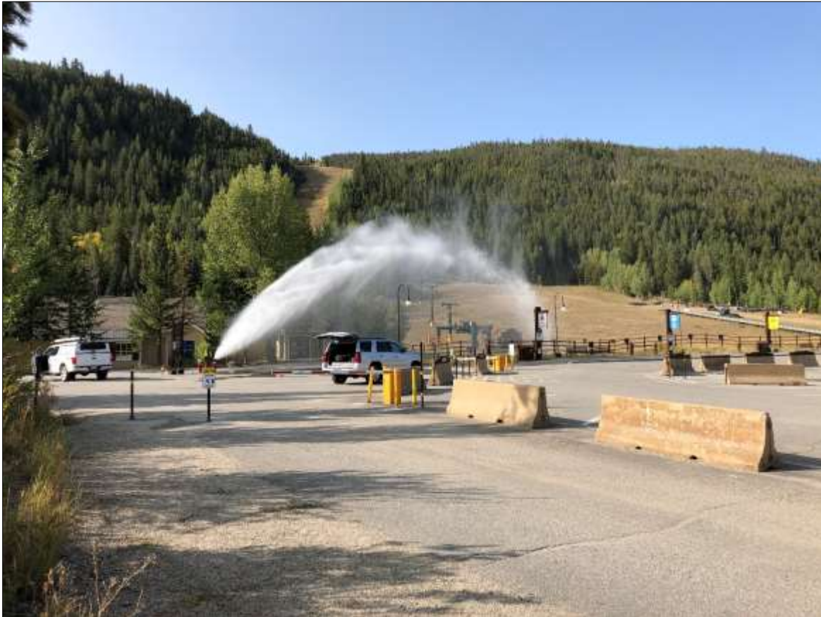
Figure 5-5 – Hydrant Flow Testing at Mountain House
